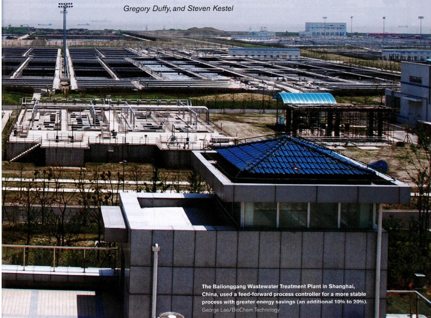
The Bailonggang Wastewater Treatment Plant in Shanghai, China, used a feed-forward process controller for a more stable process with greater energy savings (an additional 10% to 20%).
